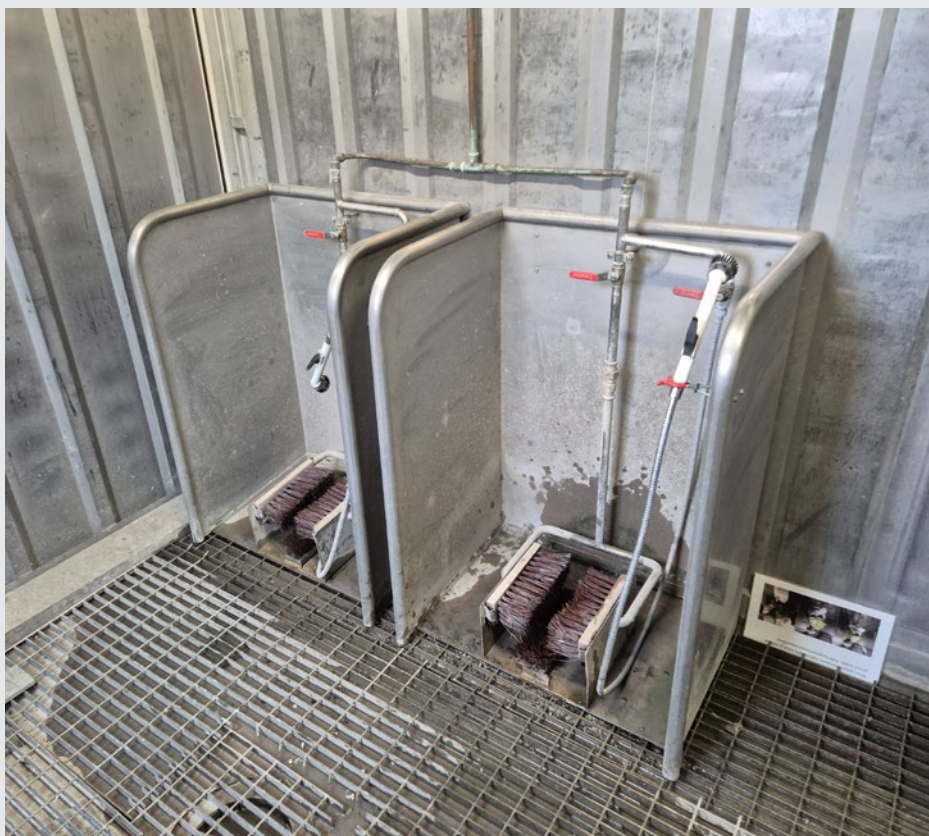
Figure 15-3: Footwear washing facilities inside a decontamination chamber
