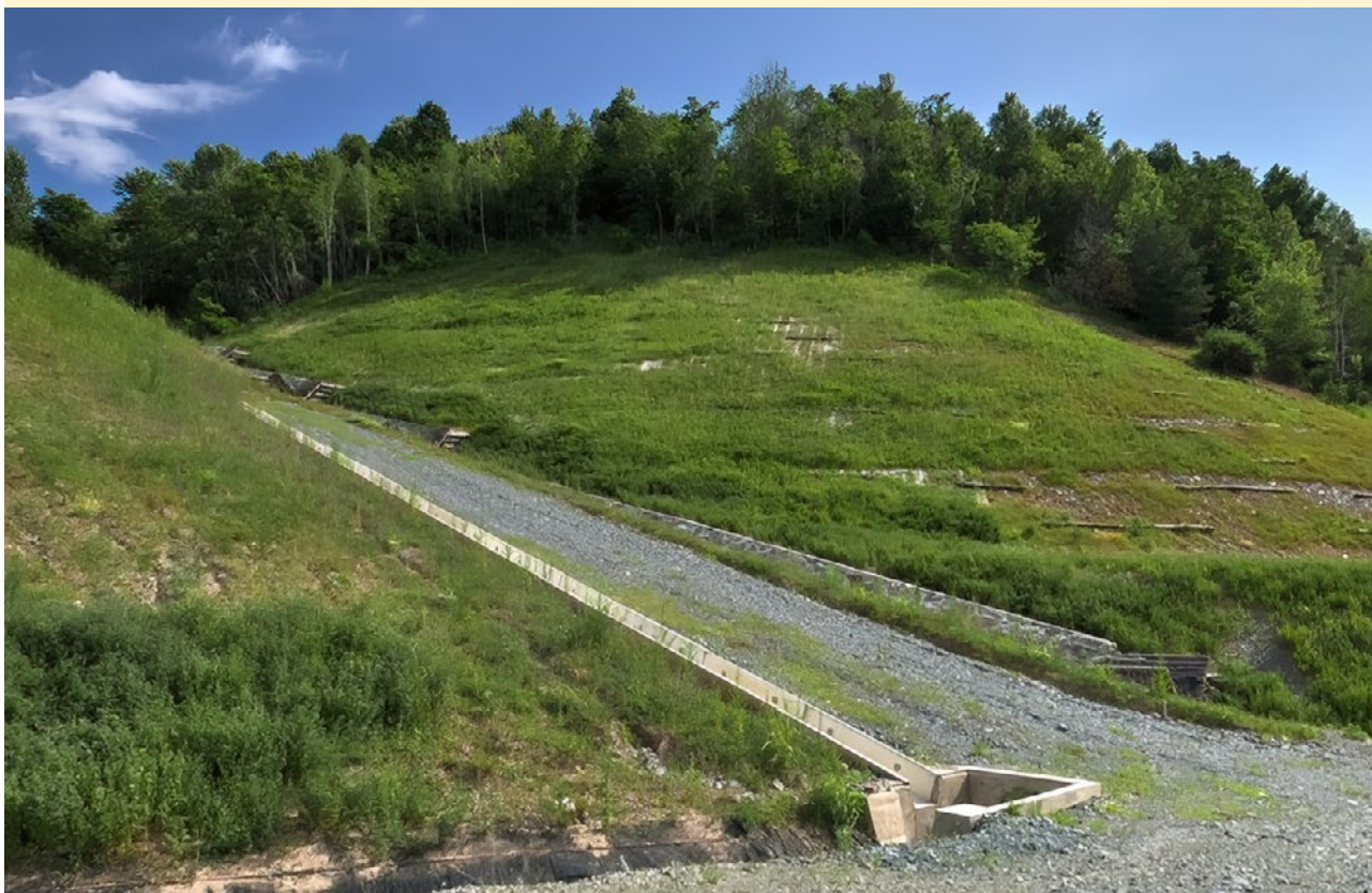
Figure 15-10: Area A after remediation: stabilised slopes covered in vegetation prevent the release of airborne dust
